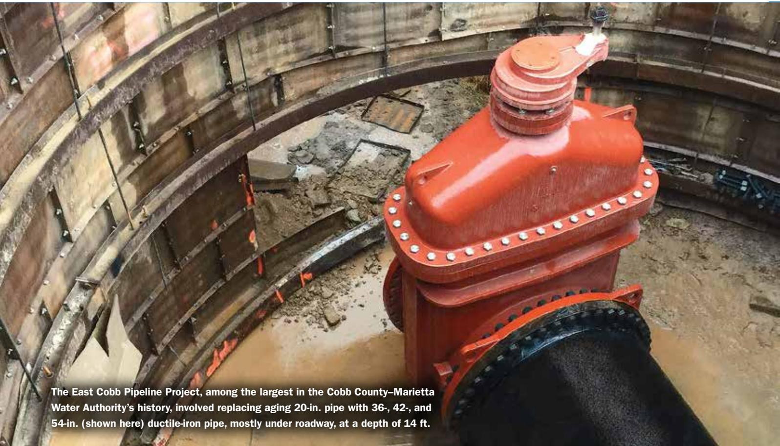
The East Cobb Pipeline Project, among the largest in the Cobb County–Marietta Water Authority’s history, involved replacing aging 20-in. pipe with 36-, 42-, and 54-in. (shown here) ductile-iron pipe, mostly under roadway, at a depth of 14 ft.
